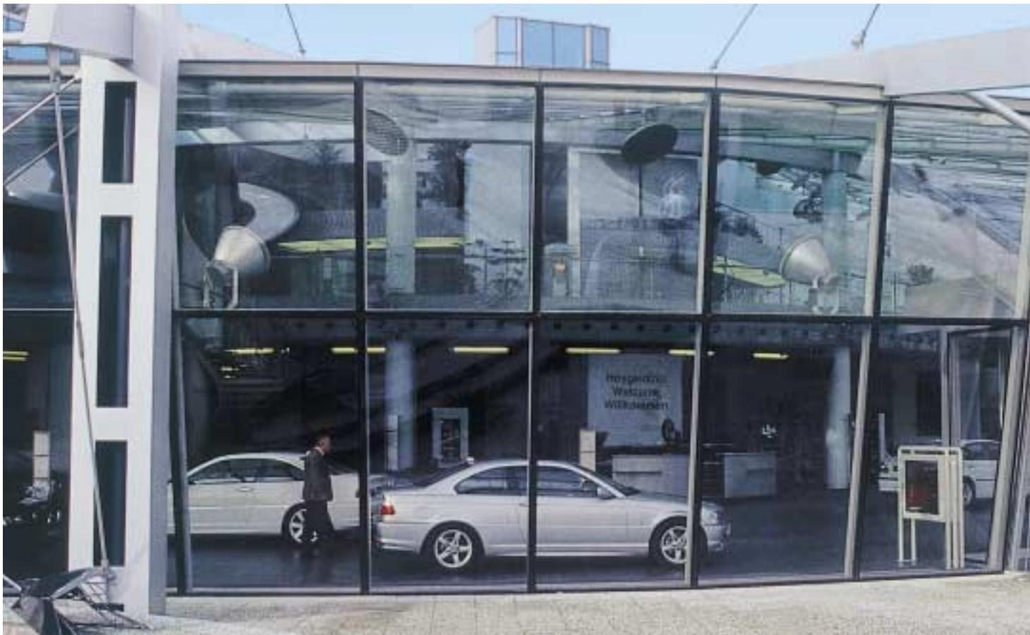
Normal glass is used in the upper section of this glass facade and AMIRAN® is used below.
